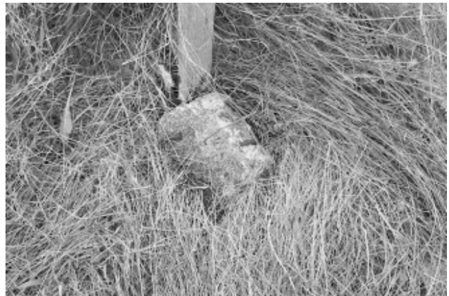
What is left of a concrete highway bound on Route 4 in Berwick, ME
